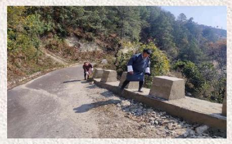
A 12 meter retaining wall was constructed at Jokai in Laptsa Chiwog and a 12.5 meter retaining wall was constructed at the Brasanma slide-prone area. This has benefitted travelers along the GC Road and reduced the incidences of accidents.
