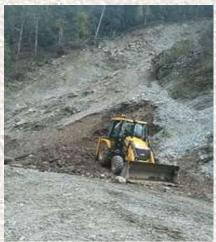
The farm roads within the Silambi Gewog constantly require maintenance, particularly because they are currently in poor condition and become especially problematic during the monsoon seasons. Heavy rainfall leads to road damage, including landslides and erosion that washes away the road's foundation, resulting in blockages for traffic. To ensure the smooth flow of traffic, it's essential to clear the blockages in the villages.
